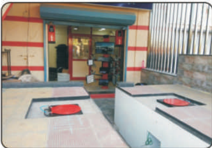
RTO office building chinchwad
